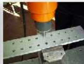
Mandrelling by using impulse riveting hammer
